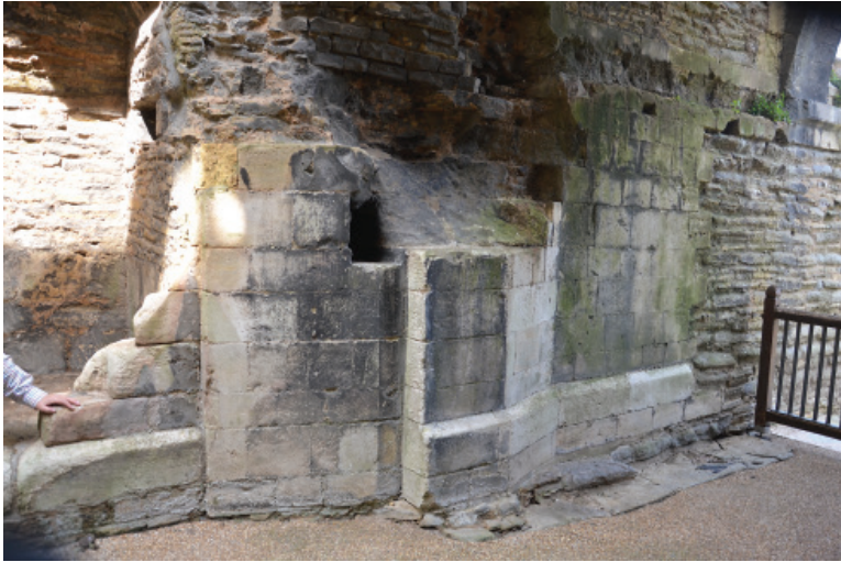
Very fine ashlar masonry of the early 12th-century gate at Newark Castle (photo J.B. Kerr)
