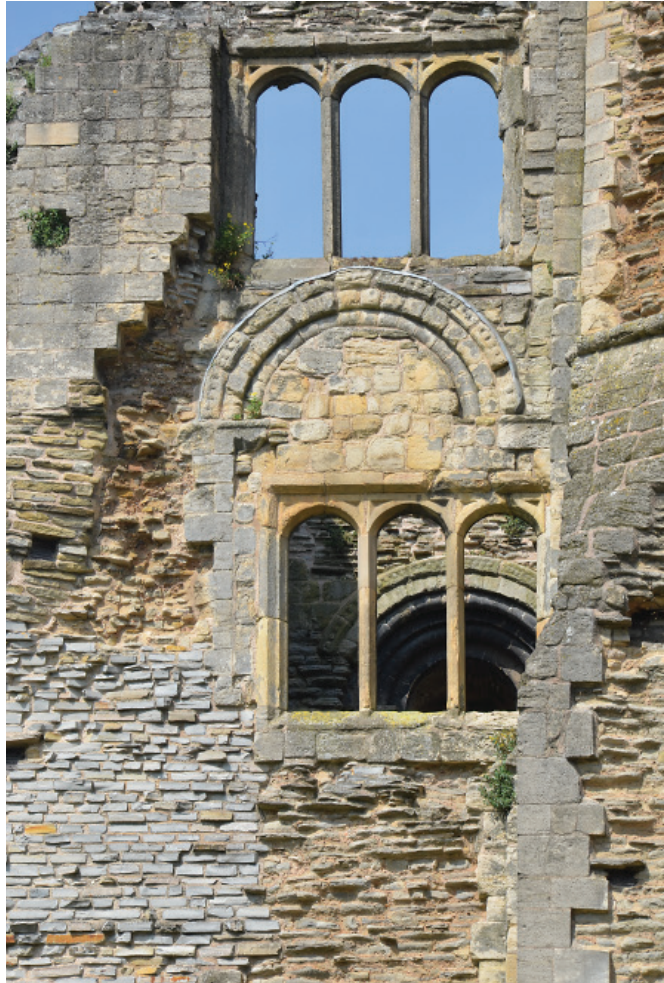
Newark Castle Gatehouse – an early 12th-century window, blocked with an inserted 16th-century window (photo J.B. Kerr)
