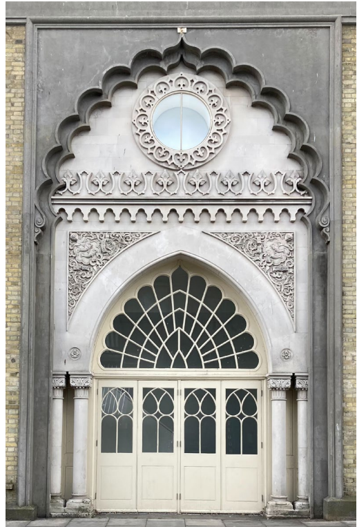
An entrance to the former Stables, now the Dome (J. Haes)
